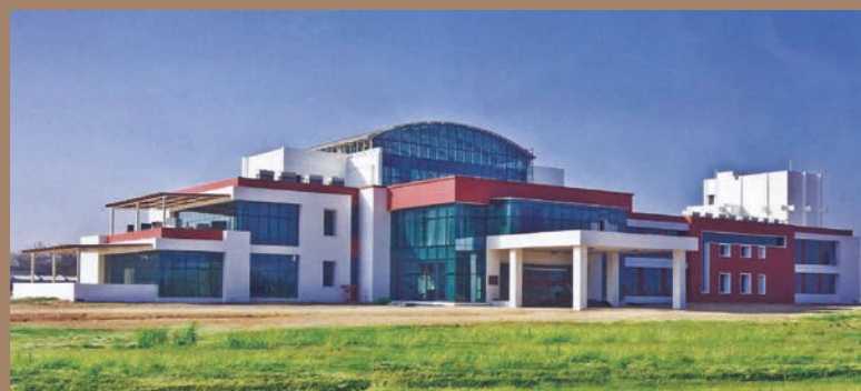
The newly constructed biotech building at ICRISAT. Photo Courtesy of Norm Weeden
