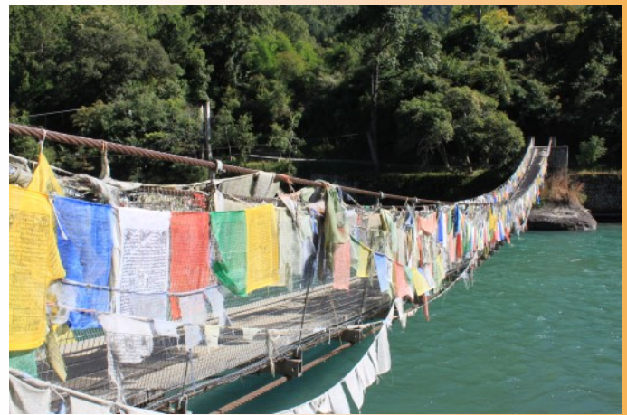
A walking bridge across Paro Chhu, in the Paro valley
